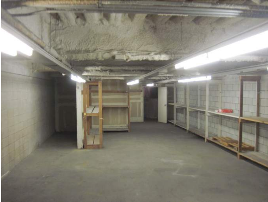
11. View of subject site ICDC College basement.
